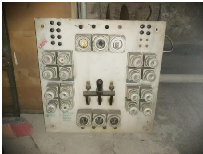
Fig. 1. Electrical panel from the years 1949-52, in an open construction
