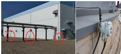
Fig. 6. Ground resistance online detector [11]
